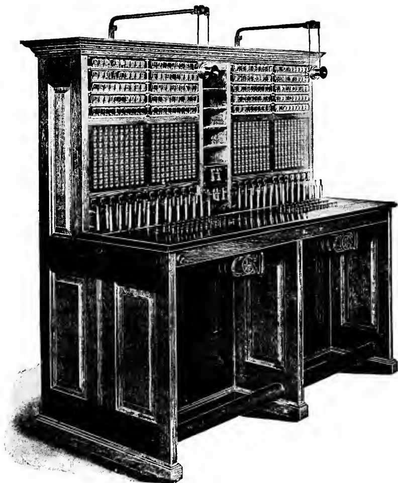
FIG. 155.—Couch & Seeley's 200-drop multiple switchboard. This cut well illustrates the multiple system, showing 400 jacks to 200 drops, or each line carrying two jacks, thus avoiding cross-connections.
